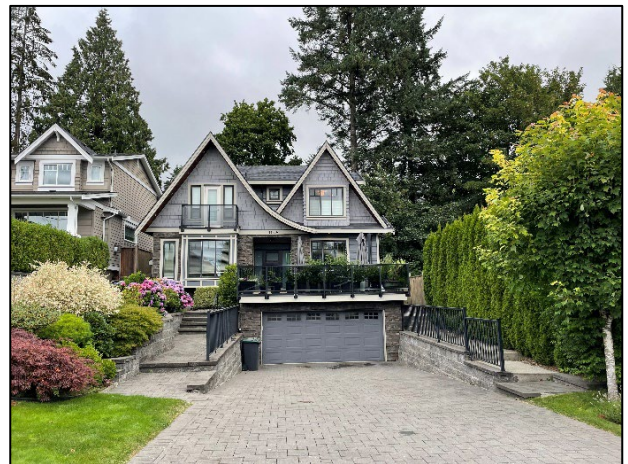
Photo 2: This garage and basement permitted under the “localized depression” rules is now permitted as a “storey” for this three-storey house.
