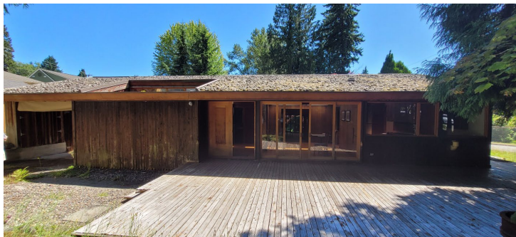
North Elevation, showing front entry, opening in the roof notes the bedroom courtyard garden.
