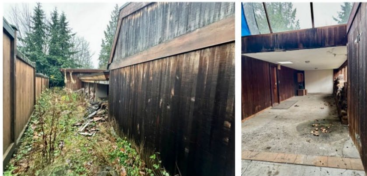
East Elevation, as is December 2025, Mountain Heritage Photo
