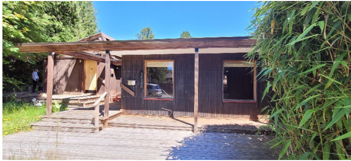
West Elevation, as seen from Everglade Place
