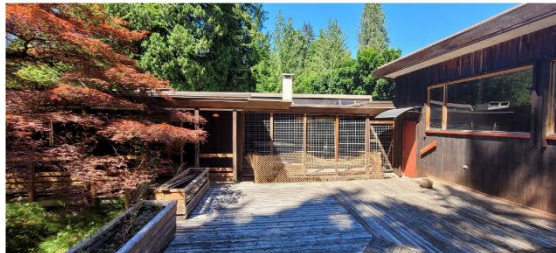
South Elevation, with garage/studio on right
