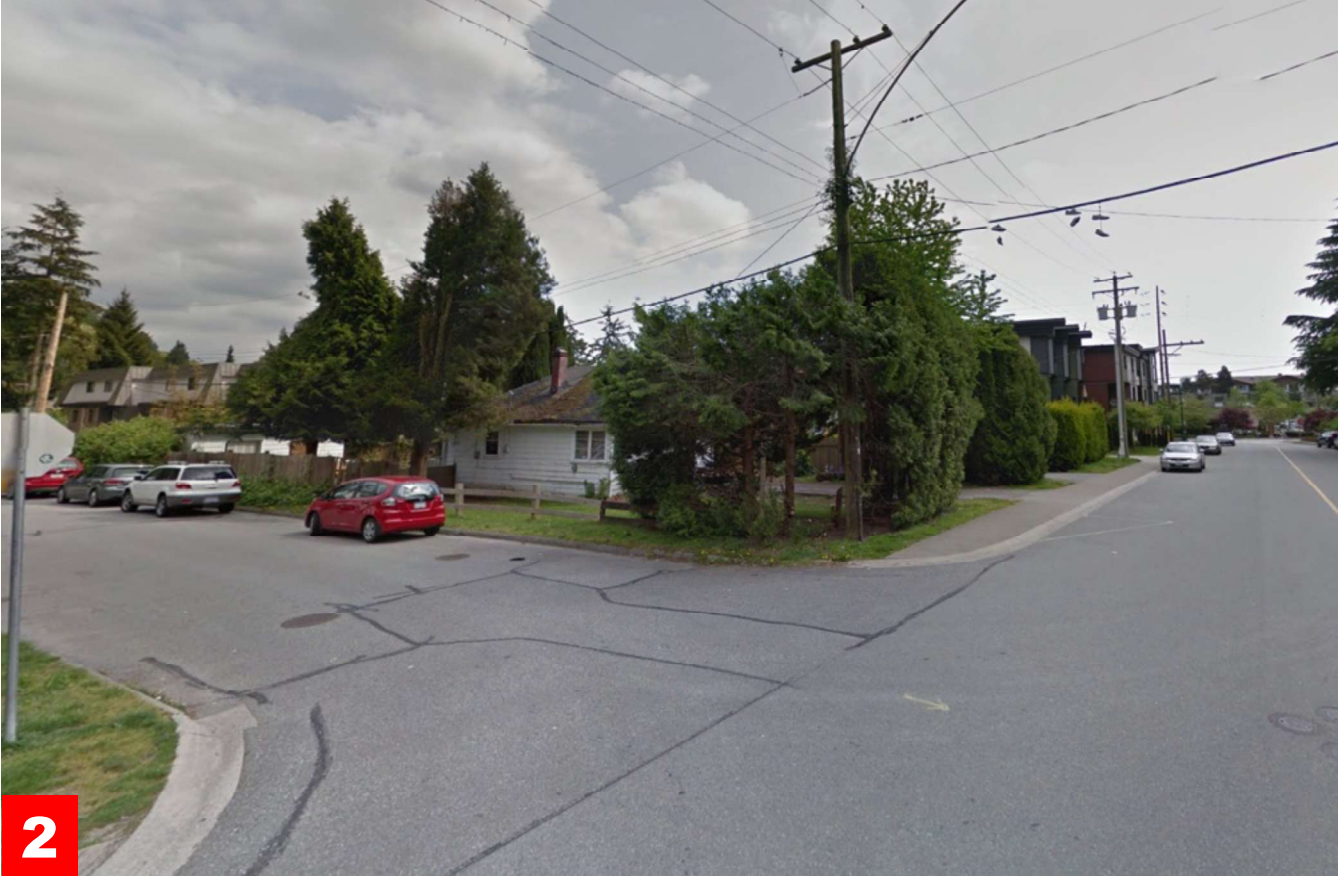
VIEW LOOKING AT NORTH-WEST CORNER
