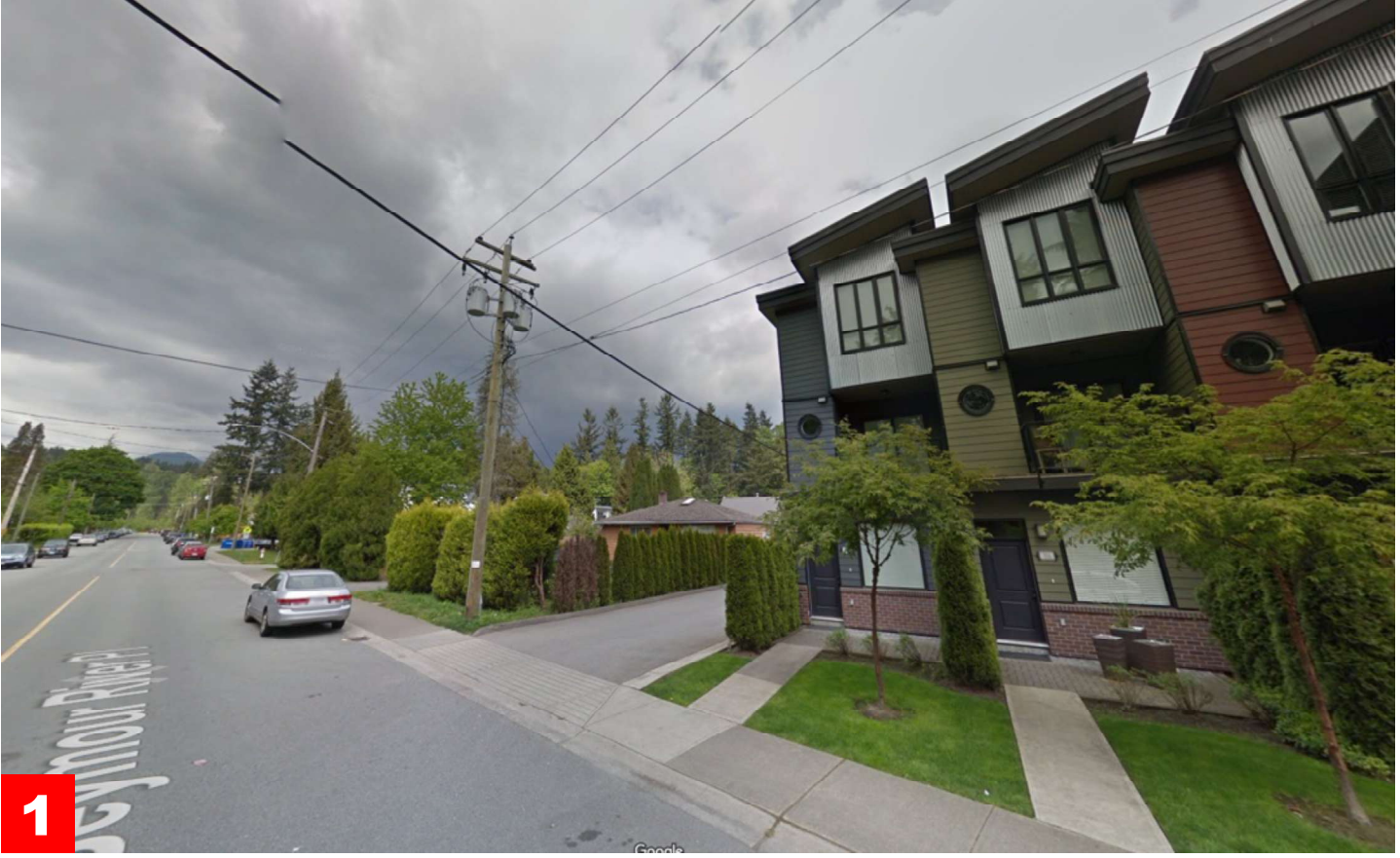
VIEW LOOKING AT SOUTH-WEST CORNER
