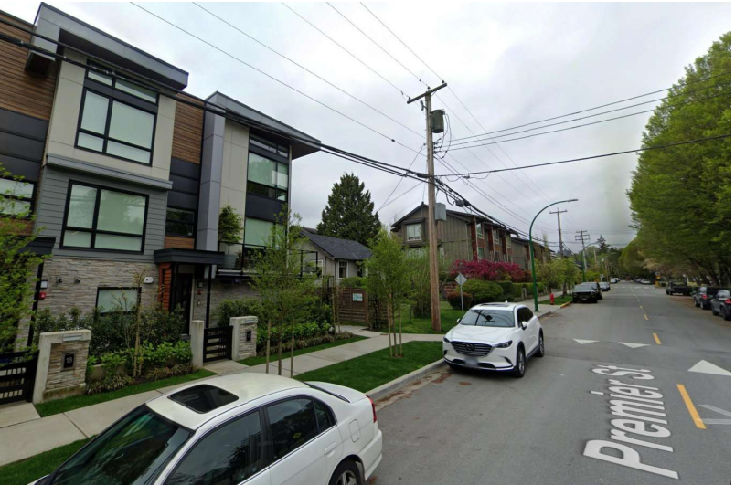
VIEW AT SOUTH-EAST CORNER
