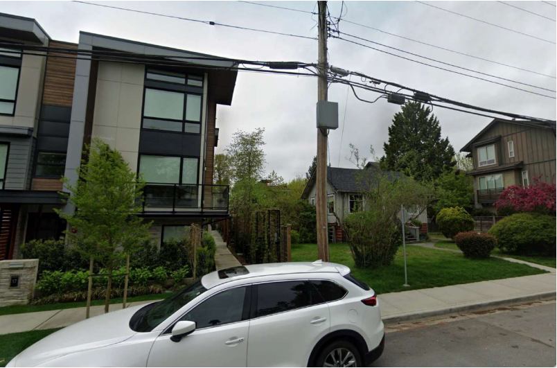
SITE VIEW LOOKING WEST
