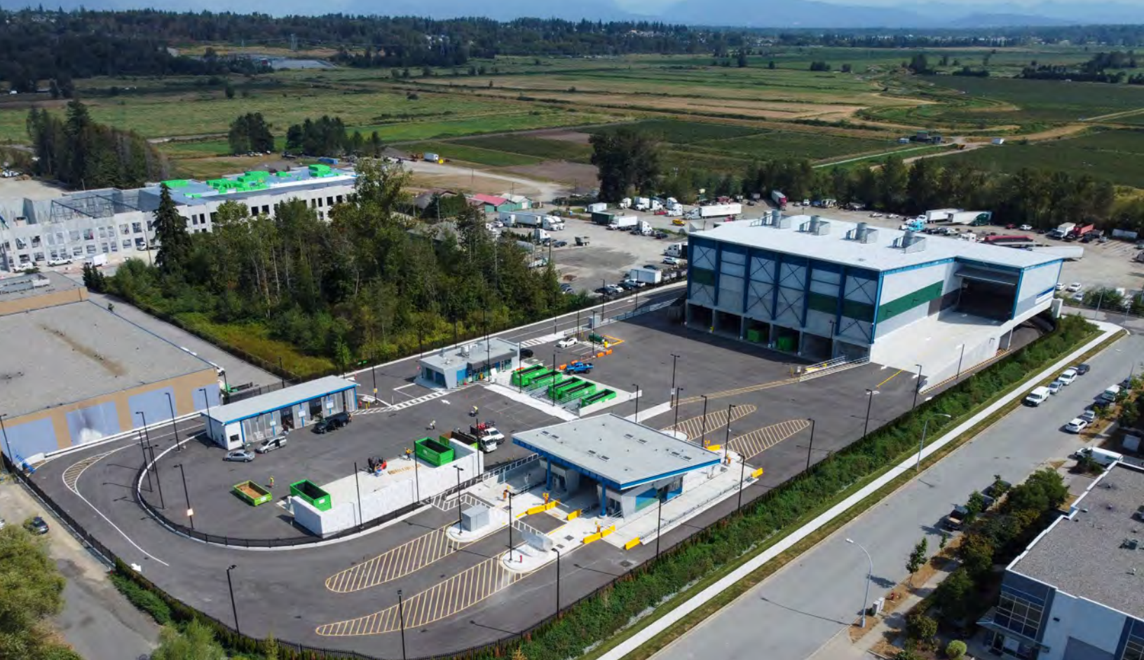
Central Surrey Recycling and Waste Centre
