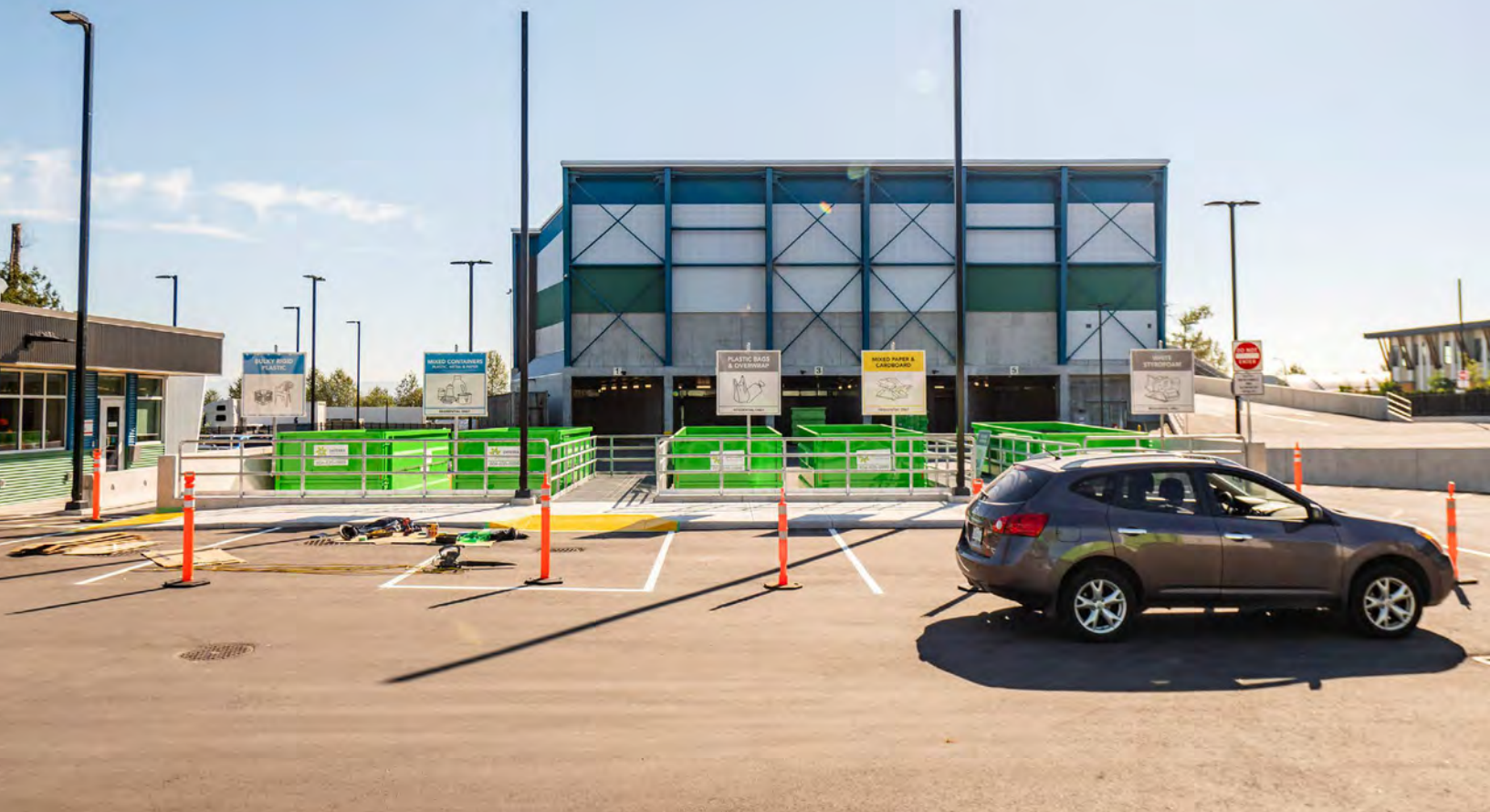
Central Surrey Recycling and Waste Center
