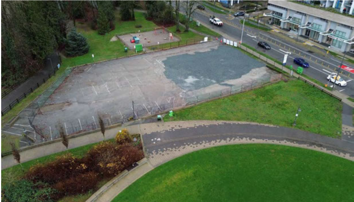
Figure 2: Seylynn Park – Existing Conditions
