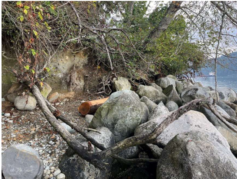
Figure 3.5 Bluff erosion with evidence of previous armoring along the west beach of WaW.
