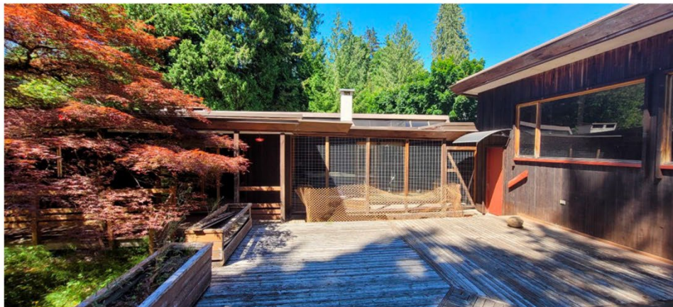
South Elevation and west elevation of studio, as is July 2025, Schueck Heritage Consulting Photo
