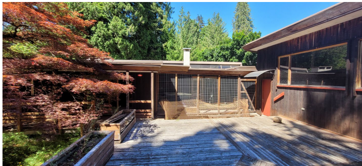
South Elevation, with garage/studio on right
