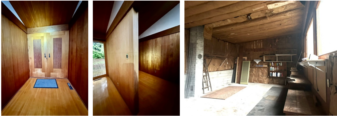
(Left to right- existing entryway, wall between existing entry way and dining area, studio)
