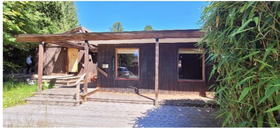
West Elevation, as seen from Everglade Place
