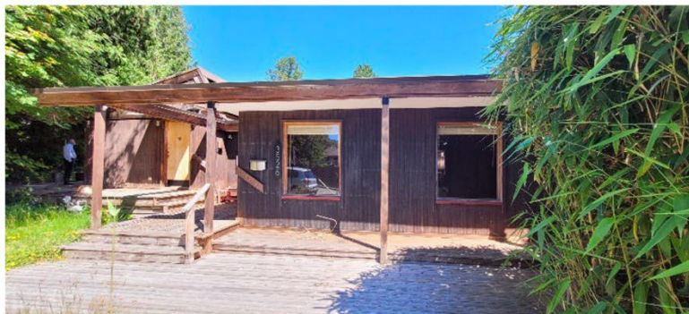
West Elevation, as is July 2025, Schueck Heritage Consulting Photo
