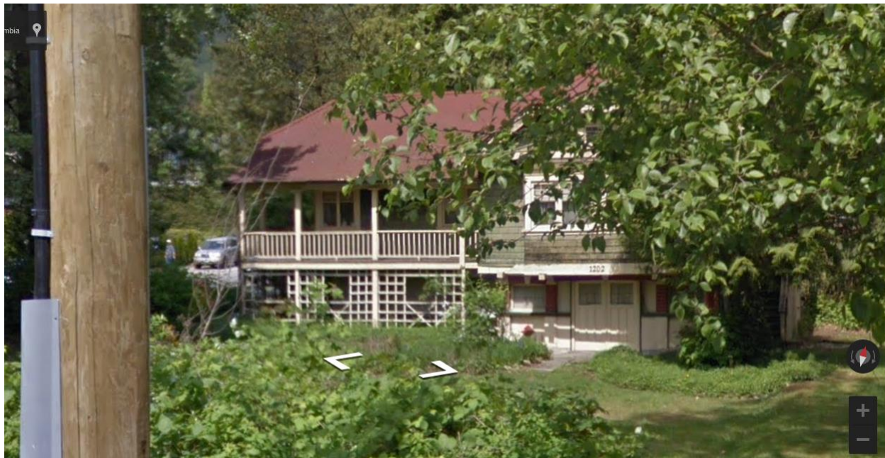
1202 Ross Road: Full south elevation, from Ross Road
