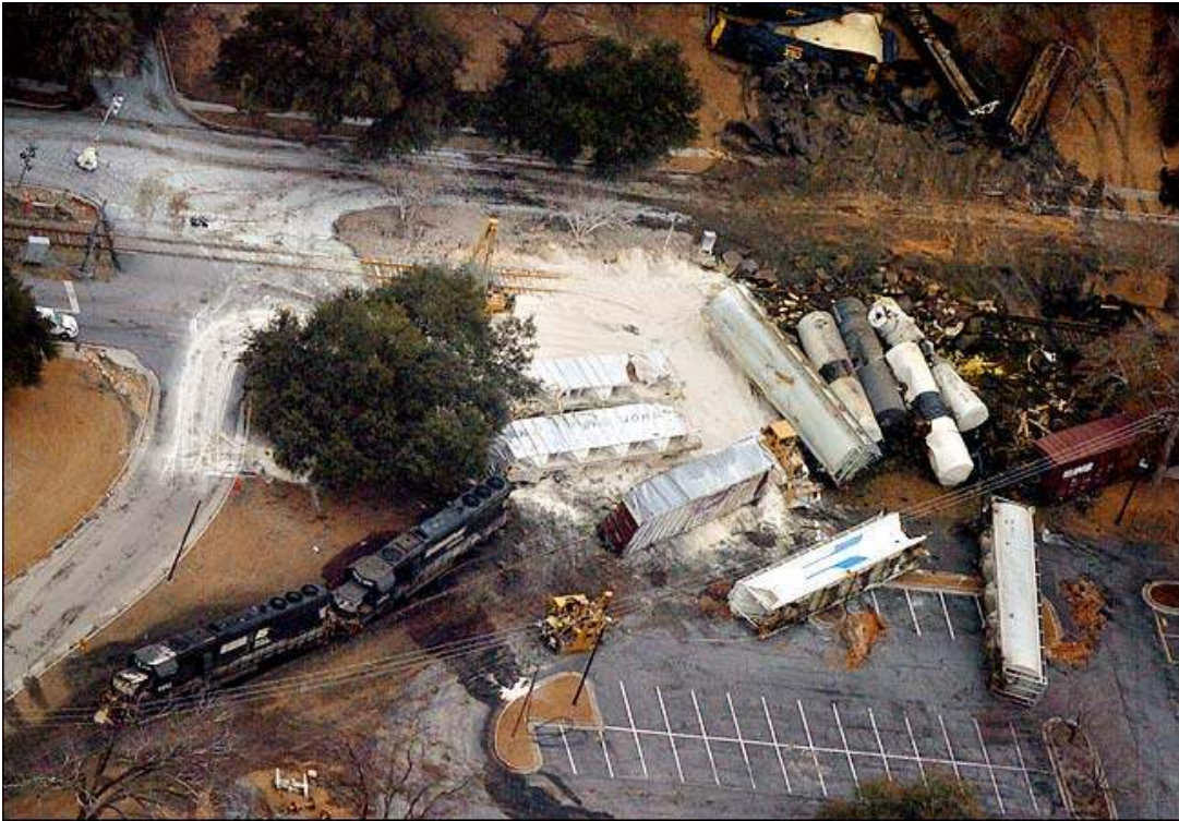
Figure 5-1: Aftermath of Graniteville, SC Incident
