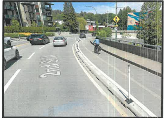
Example 3: Precast curbs with flex posts (2 nd St W, City of North Vancouver)
