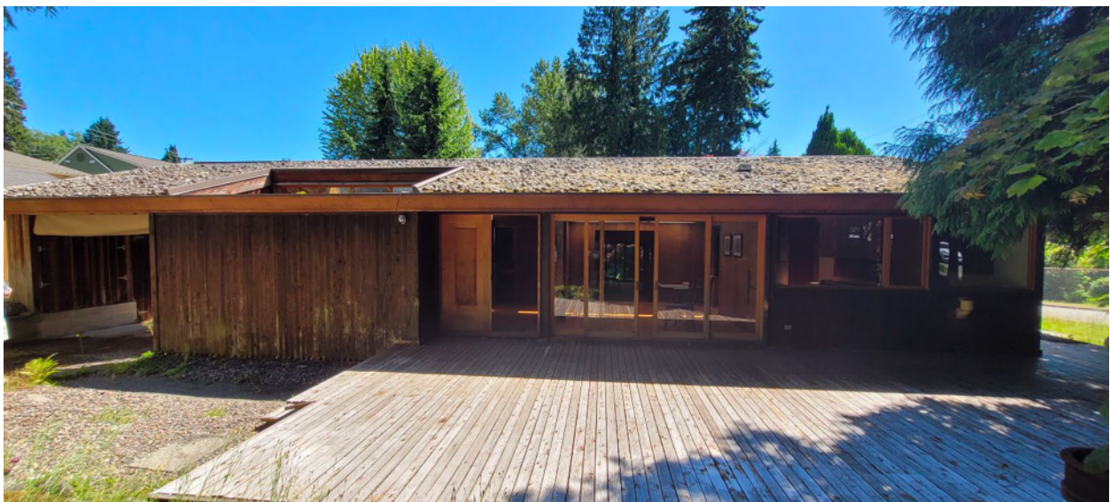
North Elevation, as is July 2025, Schueck Heritage Consulting Photo
