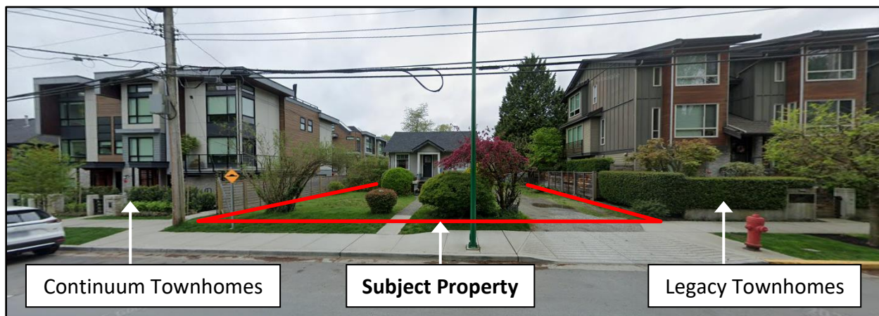
Figure 3: Existing Site Context (View Facing West From Premier Street, May 2022 Imagery)
