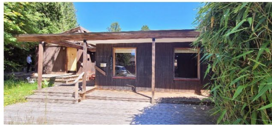
West Elevation, as seen from Everglade Place
