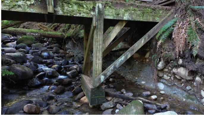
Photo 1. Northern bridge with floating footing.
