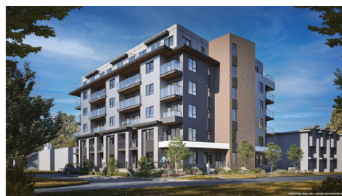
View from corner of Munster Avenue and Seymour River Place
