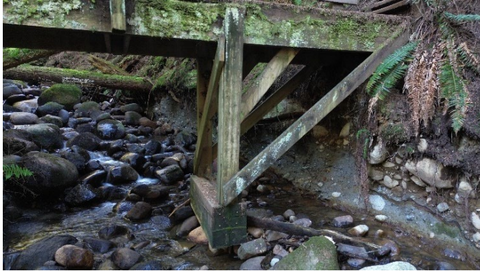
Photo 1. Northern bridge with floating footing.
