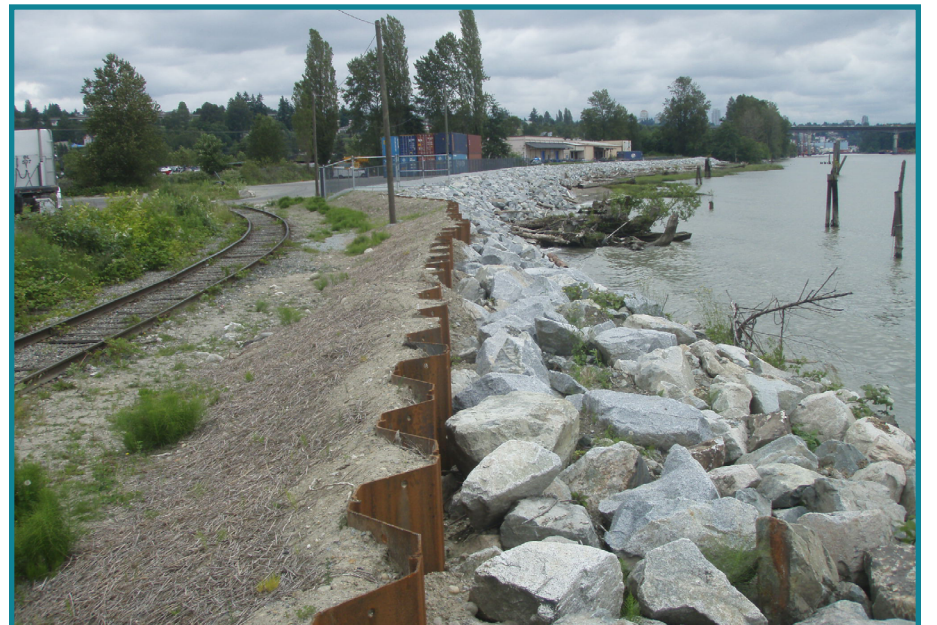
Dike made of sheet pile and rock armoring
