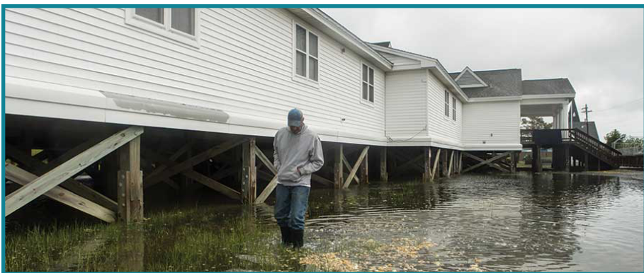
House on piles (wet floodproofing)
