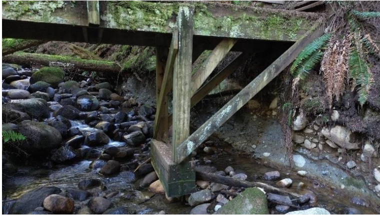
Photo 1. Northern bridge with floating footing.
